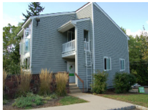
Below: Newly renovated PCNJ.
